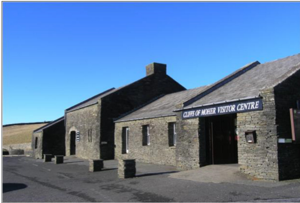
Fig. 1. Former Cliffs of Moher visitor center.
