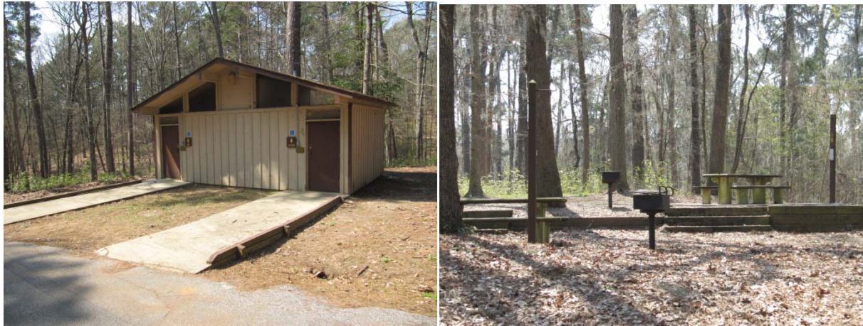
Figure 31. Ragtown, Site 18: Accessible restrooms; Camping sites
