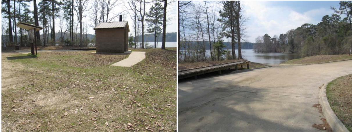
Figure 27. Haley's Ferry, Site 14: Restroom and Information board; Boat launch with access ramp
