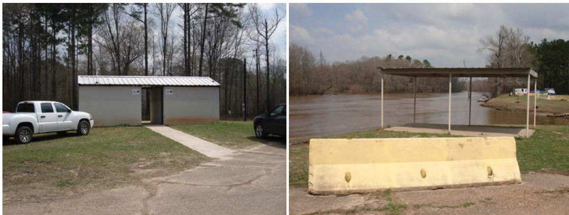
Figure 7. Garrett Park-Site 2: Restroom; Pavilion behind Jersey barrier
