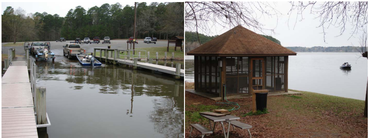
Figure 47. North Toledo Bend State Park, Site 28: Boat launch and docks; Fish cleaning station
