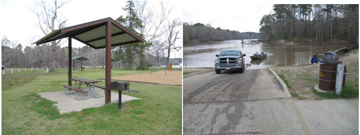
Figure 12. Swede Johnson Recreation Area-Site 4: Covered table; Boat launch ramp and trash receptacle
