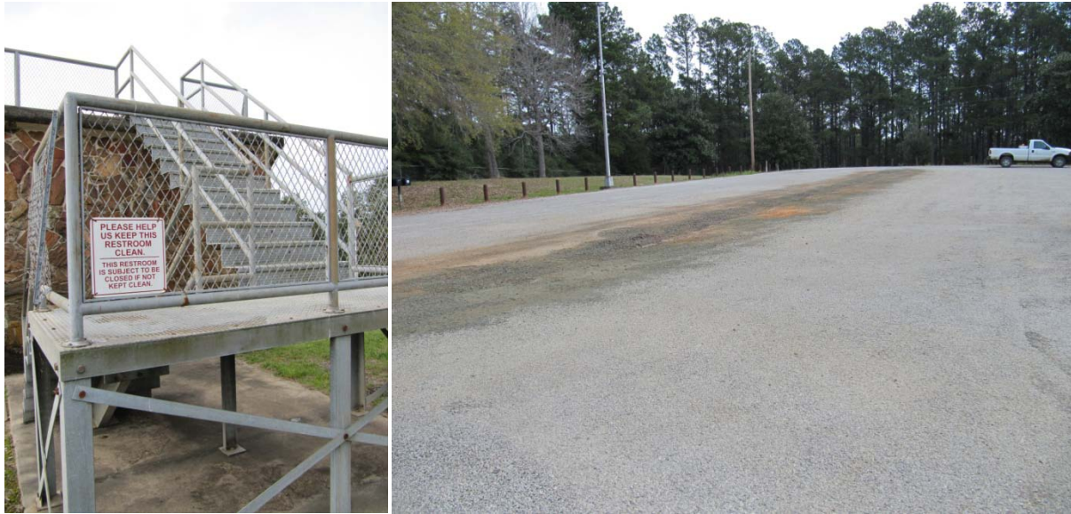
Figure 82. Dam Observation Tower, Site 79 (LA): Inaccessible route onto tower, Parking lot
