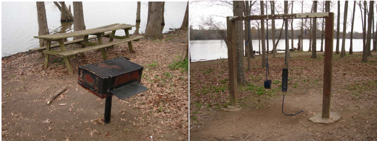
Figure 36. Clyde's Crossing, Site 21: Picnic site; Swings in disrepair
