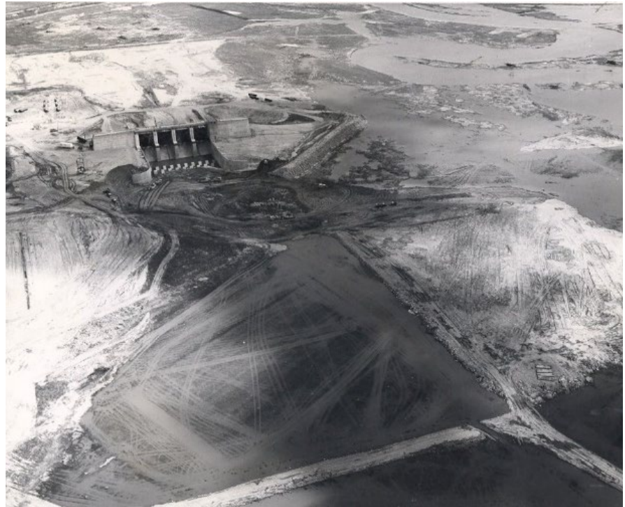
Figure 2.3.1. Construction of the Carlyle Dam, 1967
